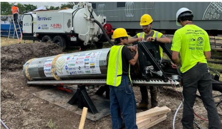
(Preparing the Launch Stand)
