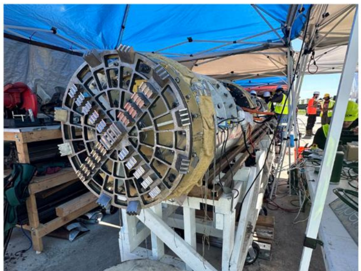
(TBM on Day 3 Prepared for Safety Check Inspections)
