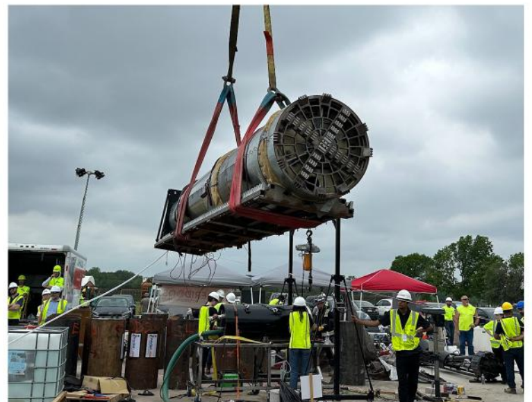
(TBM Being Lifted to its Launch Position)
